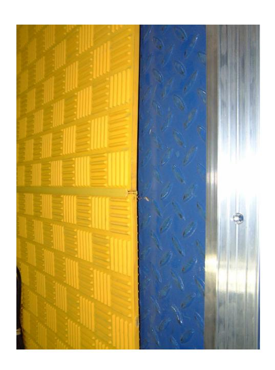
The surface of the Safety Mat will be bowed up Slightly as a result of the Active Uniting Trim sitting beneath it.
