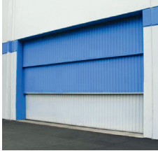
Figure 1: Typical GridScan/Pro SI application environments
